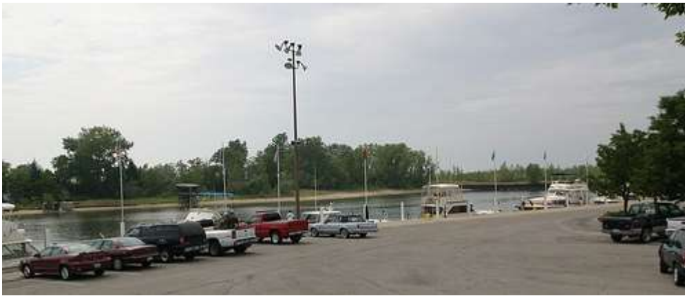
Seawall along the Trail Creek just outside the Washington Park Marina.
