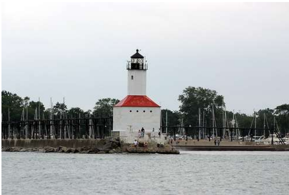
Lighthouse at the entrance to the Washington Park Marina.
