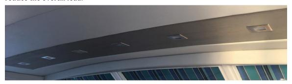
Many of the new lights are normal household fixtures fitted with 12V dimmable LED bulbs, driven by Anigmo dimmers and operated by Vimar Elkon switching. I include the details here because determining what actually works together well is harder than you might think.
