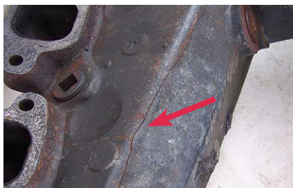
Even a short freeze can cause expanding ice to crack a manifold.
