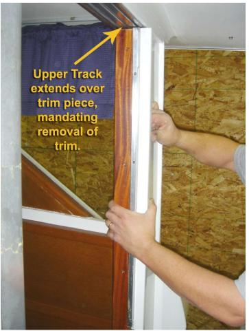
Removal of vertical trim piece not required on all boats. If upper track does not extend over the vertical trim piece, this step not required ©
