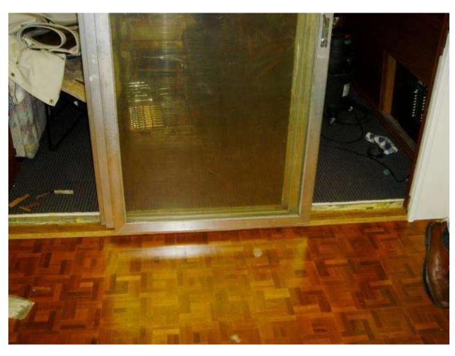
Pulling sill plate loose after cutting the sealant away. While optional, this gives more room to handle doors & upper track assembly.
