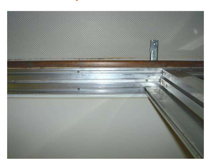
Slide doors to area you have removed screws from and take weight off of track by prying from below as shown.
