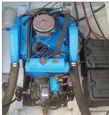
The boat was repowered with a rebuilt GMC 305 (5-liter) V-8 and a ZF Hurth HSW-450 transmission. Note the refinished hull interior. It's easy to spot dropped parts or fluid leaks in a white bilge.
