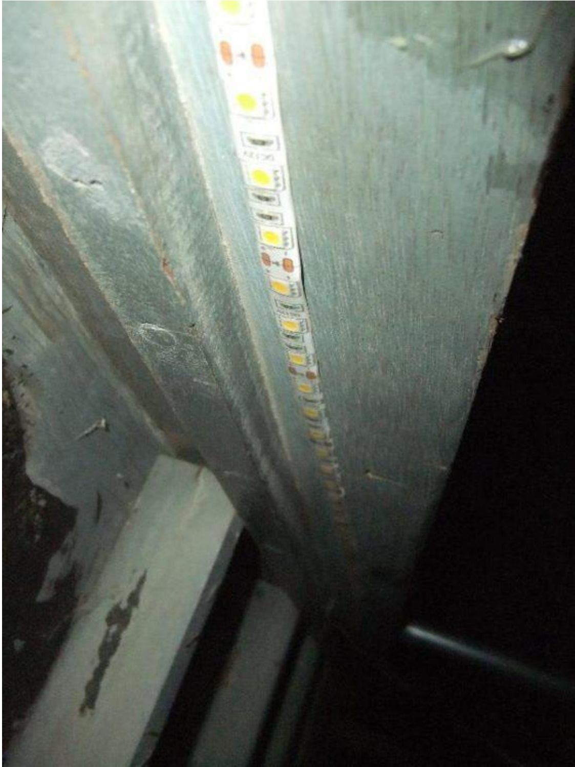
Wipe the attachment area clean and firmly press the LED in place
